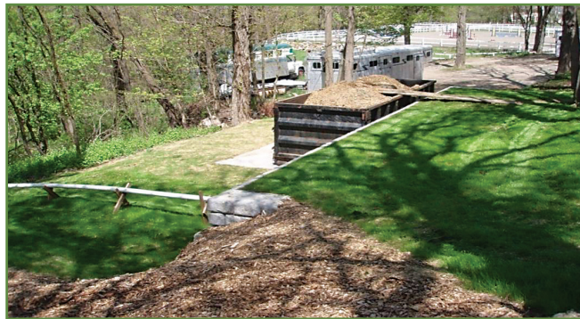
After receiving assistance and funding from the Council, this farm's revised waste system now includes a retaining wall, convenient and safe dumpster access, and concrete pad that minimizes water quality issues, improves hauling access and ultimately saves the farm money.
