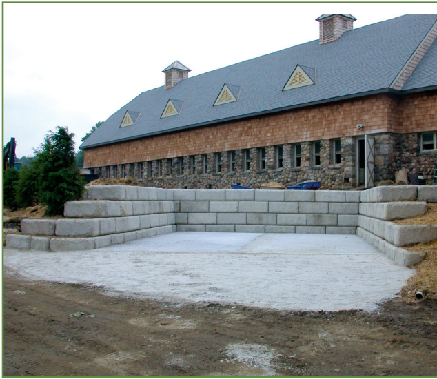
Concrete storage pads located away from water courses provide temporary manure containment until farm waste is hauled away, composted or disbursed according to a nutrient management plan.
