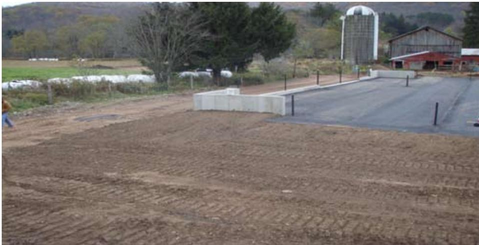
The team designed a barnyard feeding area with water management system and laneway improvement (pictured at left). Because of the herd size, the team felt a harder surface was appropriate. Barnyard clean-up would be easier on an asphalt surface compared to gravel (the traditional barnyard option for beef operations), but less
